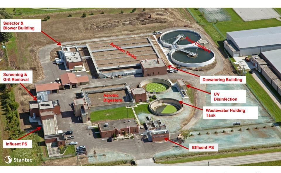
The treatment plant was designed for an average daily sewage flow of 14,500 m<sup>3</sup>/d and a peak flow capacity of 35,069 m<sup>3</sup>/d.
